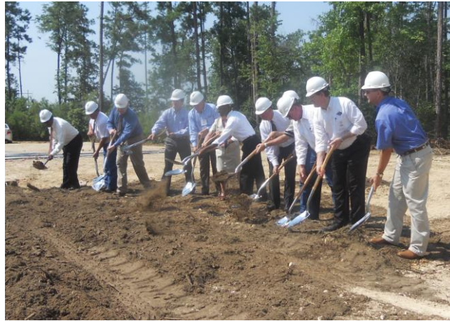
Elected Officials and Electric Cooperative Representatives Break Ground for the Woodville Renewable Power Project
